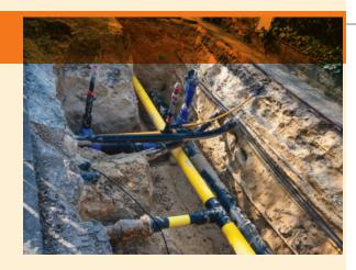
kind of damage can happen during digging or excavation. The EFV is installed underground on the service pipeline that runs between the natural gas main (usually near the street, alley, or easement) and the Avista meter on the customer's property. Typically, the EFV is installed as close as possible to the natural gas main.
