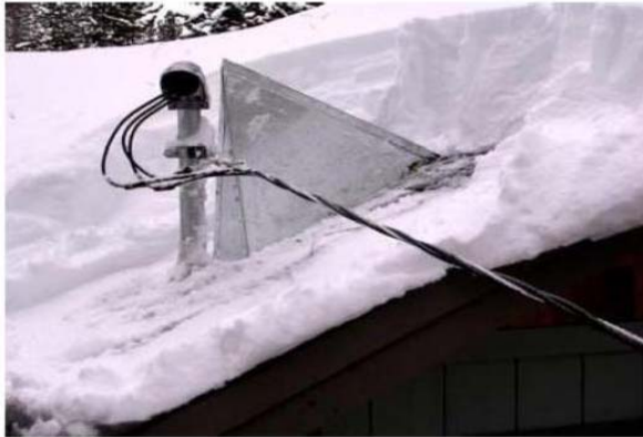
Snow Splitter constructed out of sheet metal are an alternative to Roof Crickets when only the mast needs to be protected.
