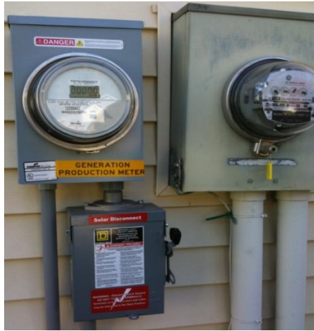
Figure 38 – Generation Production Meter and Disconnect Location
