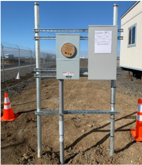
Figure 18 – 200 A Pipe Meter Pedestal Install Photo
