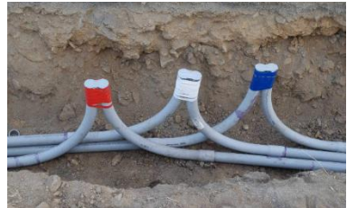
Figure 26 – Conduit Entrance 3-Phase Padmounted Junction Enclosures
