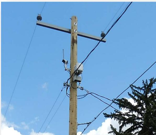
*The combination of wood poles with fiberglass crossarms rarely cause pole top fires. This is a proven tactic for reducing the risk of utility involved fires and is a component of distribution grid hardening.*
