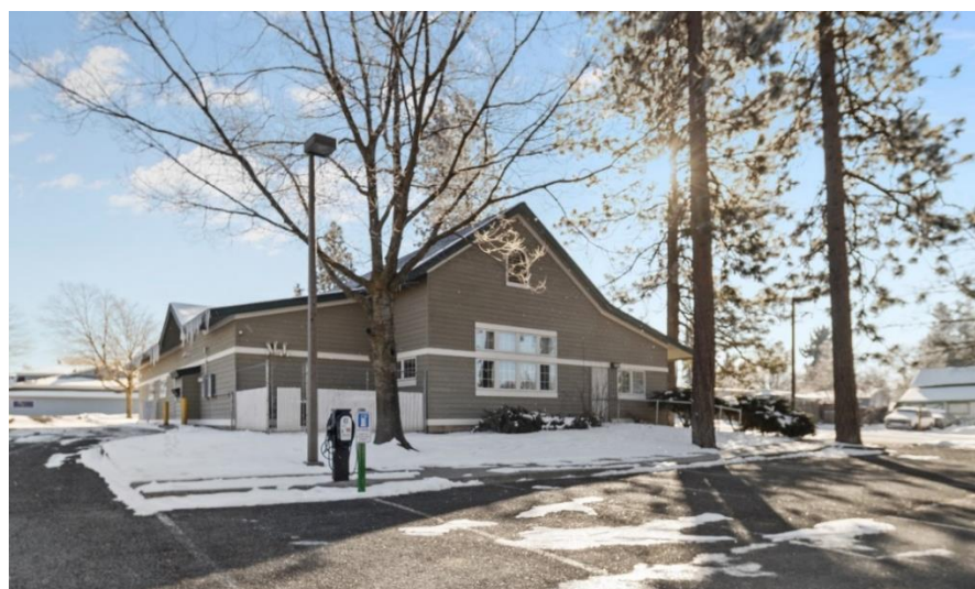
Figure 9: Community public charging installation at the Medical Lake Library
