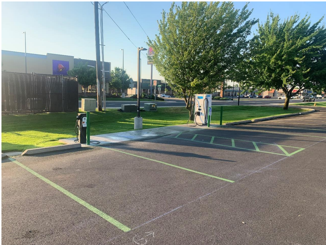
Figure 11: Yokes Fresh Market Deer Park Charging Station
