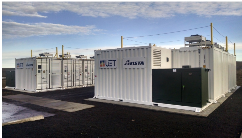
Turner Energy Storage Project, Pullman, WA
