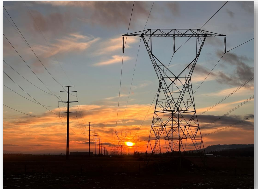
Avista's 230 kV (left) and BPA's 230 kV line across the Rathdrum Prairie, ID
