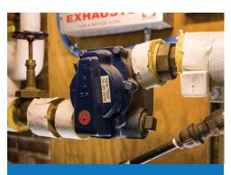
A rebuilt steam trap.
