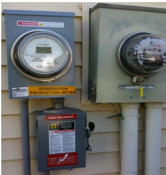
Figure 6.1 – Generation Production Meter and Disconnect Location
