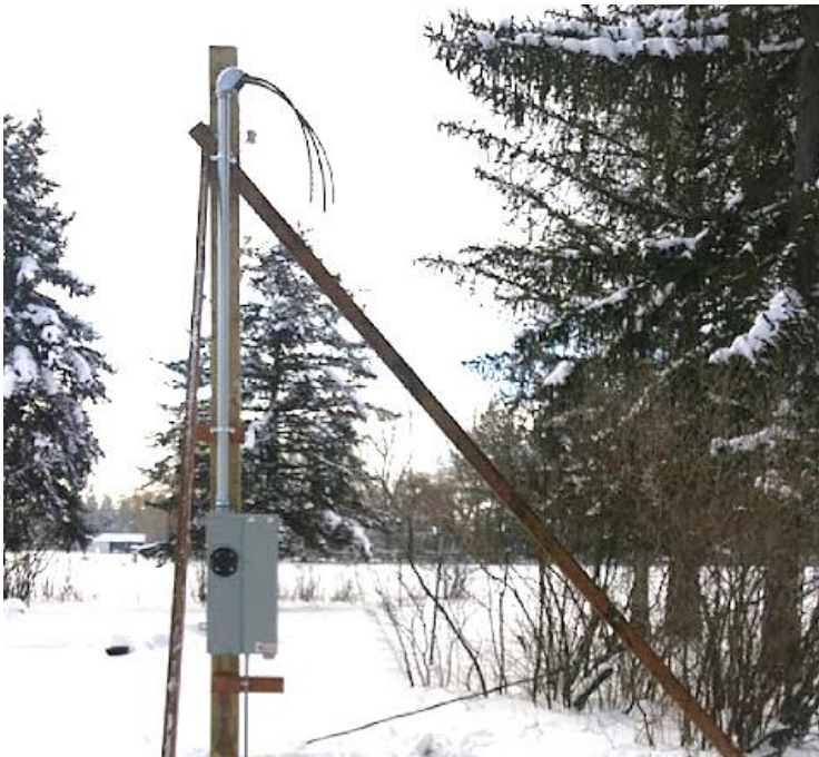
Figure 2.1 – Temporary Overhead Service
