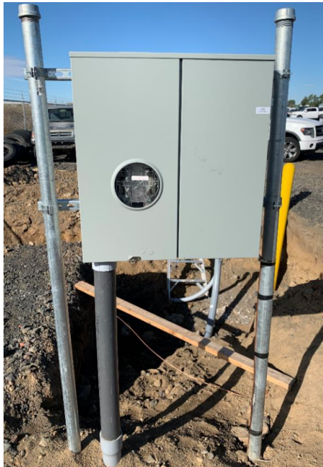
Figure 4.17 – 400A Pipe Meter Pedestal Install Photo
