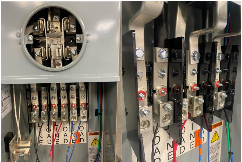
Figure 5.2 – Safety Socket Bypass
