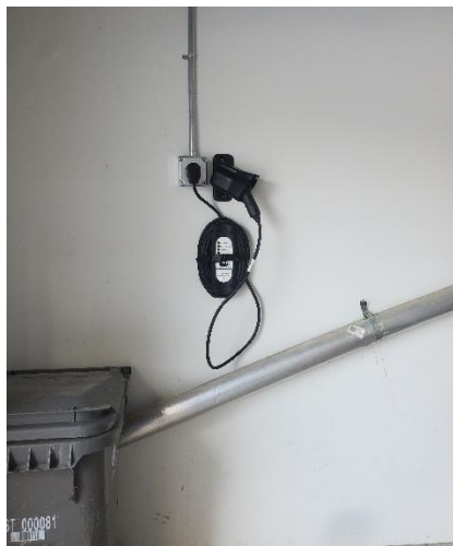
Figure 5: Residential charger installation
