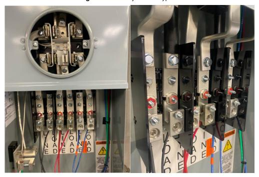
Figure 5.2 - Safety Socket Bypass
