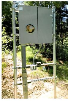
Figure 4.18 – Pedestal Mounted CT Enclosure Install Photo
