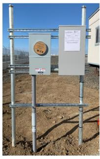
For residential only, a wood post embedded in concrete may be used for 200A meter pedestal in lieu of the rigid steel pipes and unistrut. Wood posts must be either a commercially new  $6'' \times 6''$  treated post or a minimum 8-inch top diameter butt treated cedar or full treated white wood pole as depicted below.
