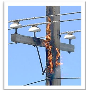
Figure 12. Pole fire associated with wood crossarm
