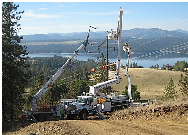
Figure 29. Addy-Gifford Steel Pole Replacement Work
