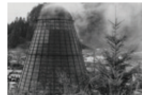
Decades ago, sawmills would burn their own waste in large wigwam burners, generating a consistent blue haze every morning before the fires heated up.
